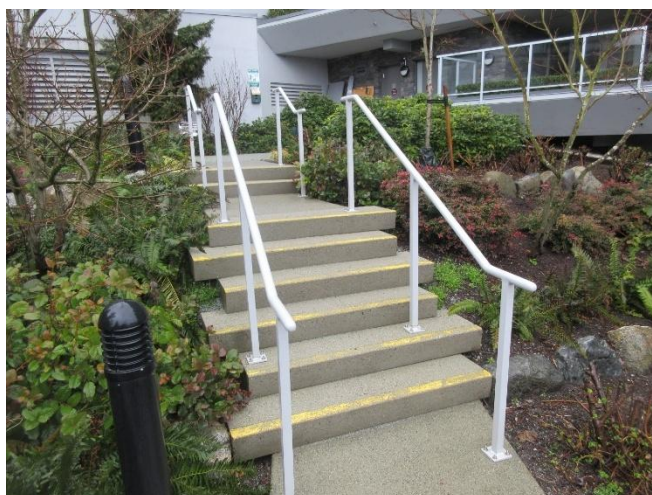
Photo 25: Concrete stairs, railings and soft landscaping.
