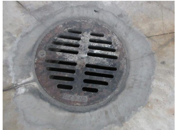
Photo 37: Typical catch basin.
