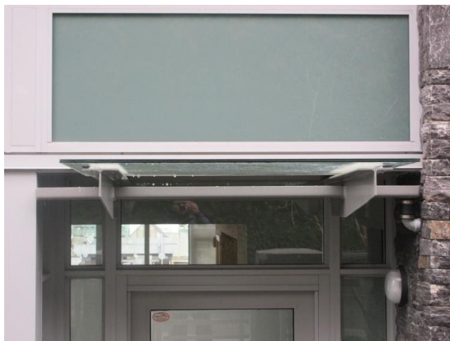
Photo 8: Typical metal canopy over townhouse unit entrance.
