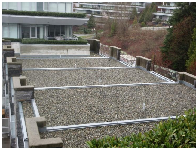
Photo 14: Ballasted roofs over the townhouses.
