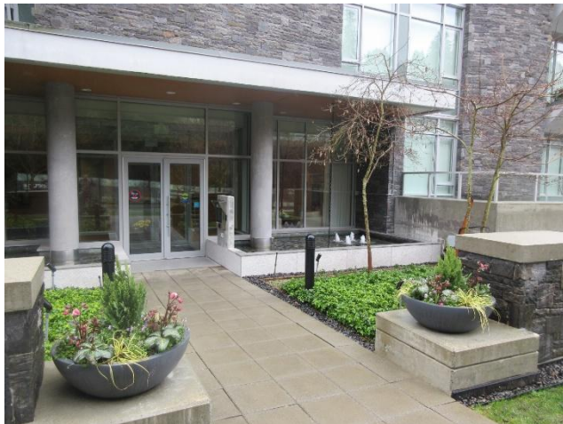
Photo 1: Typical building entrance.
