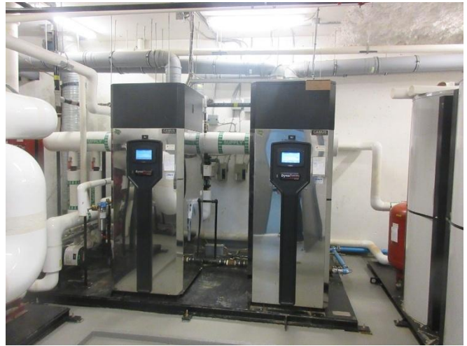
Photo 27: Heating boilers.
