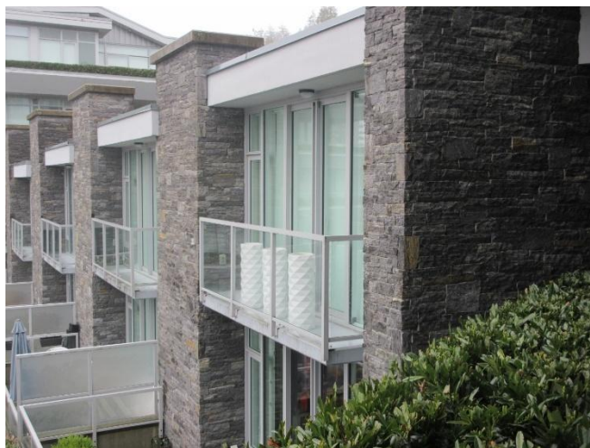
Photo 3: Typical townhouse unit balconies.
