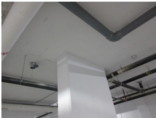
Photo 1: Typical structure in the parking garage.
