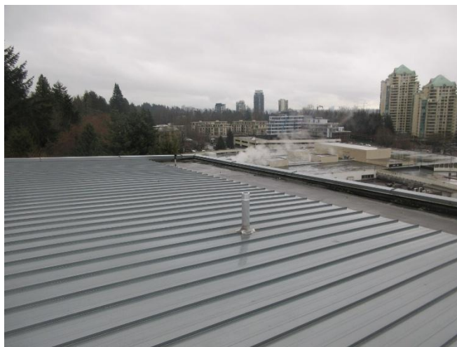
Photo 13: Typical sloped metal and exposed bitumen roof.
