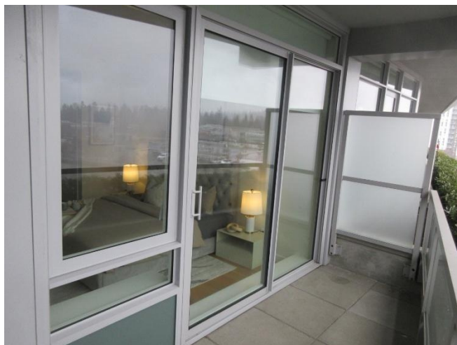
Photo 10: Typical single sash sliding door.
