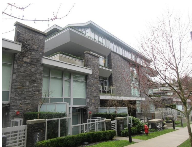
Photo 7: Typical exterior walls.
