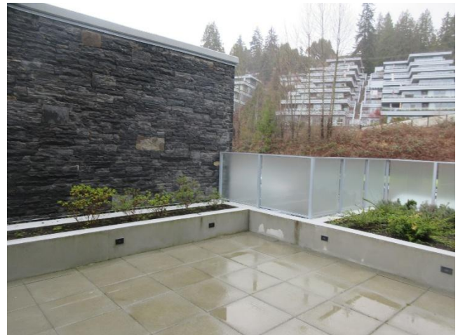
Photo 2: Typical site features and paving.
